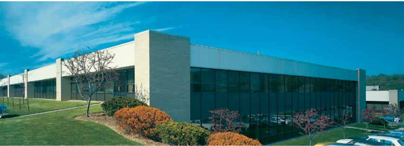
These versatile buildings feature separate office entrances and hidden rear loading courts.
